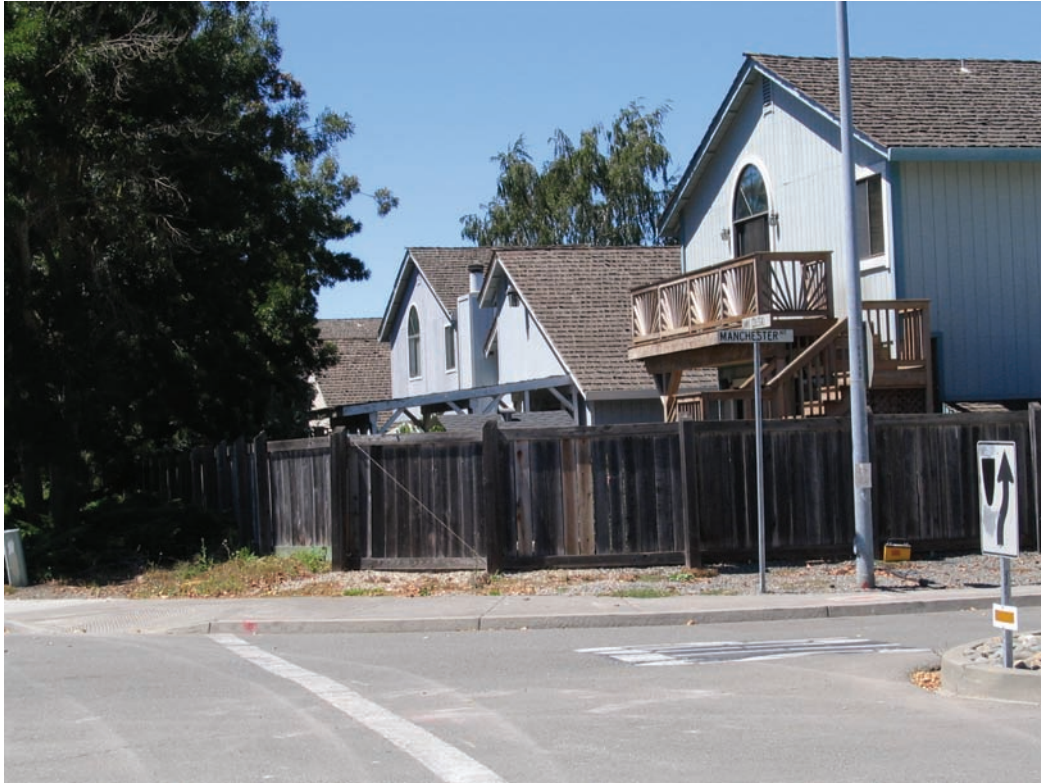
A. Homes fronting Camino Collegio (North side, west of Manchester Avenue) – Wood fence only.
